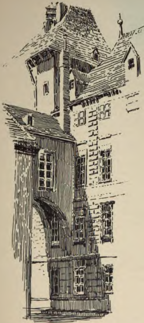
BRIDGE CONNECTING THE OLD BALLHAUS WITH THE HOFBURG ( now demolished )
